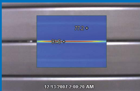
In a data centre with a conditioned airflow temperature of 72°F (22°C), and a series of non-HotLok Blanking Panels installed, the measured temperature of the heat radiating through the horizontal gaps is 91.5°F (33°C), which is much higher than the ASHRAE - recommended 77°F (25°C).
