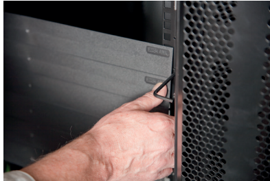
Place the panel in the required position & align the clips with 19" mounting holes
