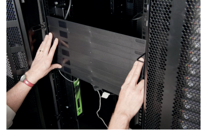
Push the clips firmly into position on each side
