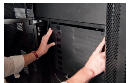
Insert the adjusted panel to fill the remaining open rack space.
