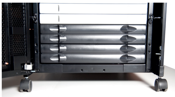
Rack With No Seal Air can freely flow under rack
