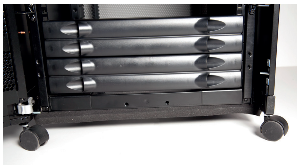
RackSEAL Applied To Base of Rack Once applied barrier starts to expand
